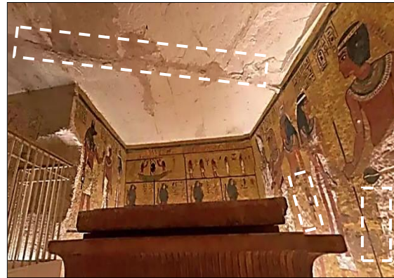
Figure (7) laminar peelings resulting from internal stress
